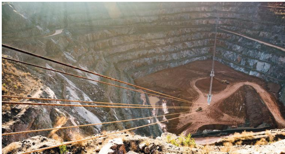
The Doppelmayr RopeCon solution at Bardon Hill Quarry transports up to 1,000 tonnes of overburden per hour, reducing environmental impact and CO 2 emission
