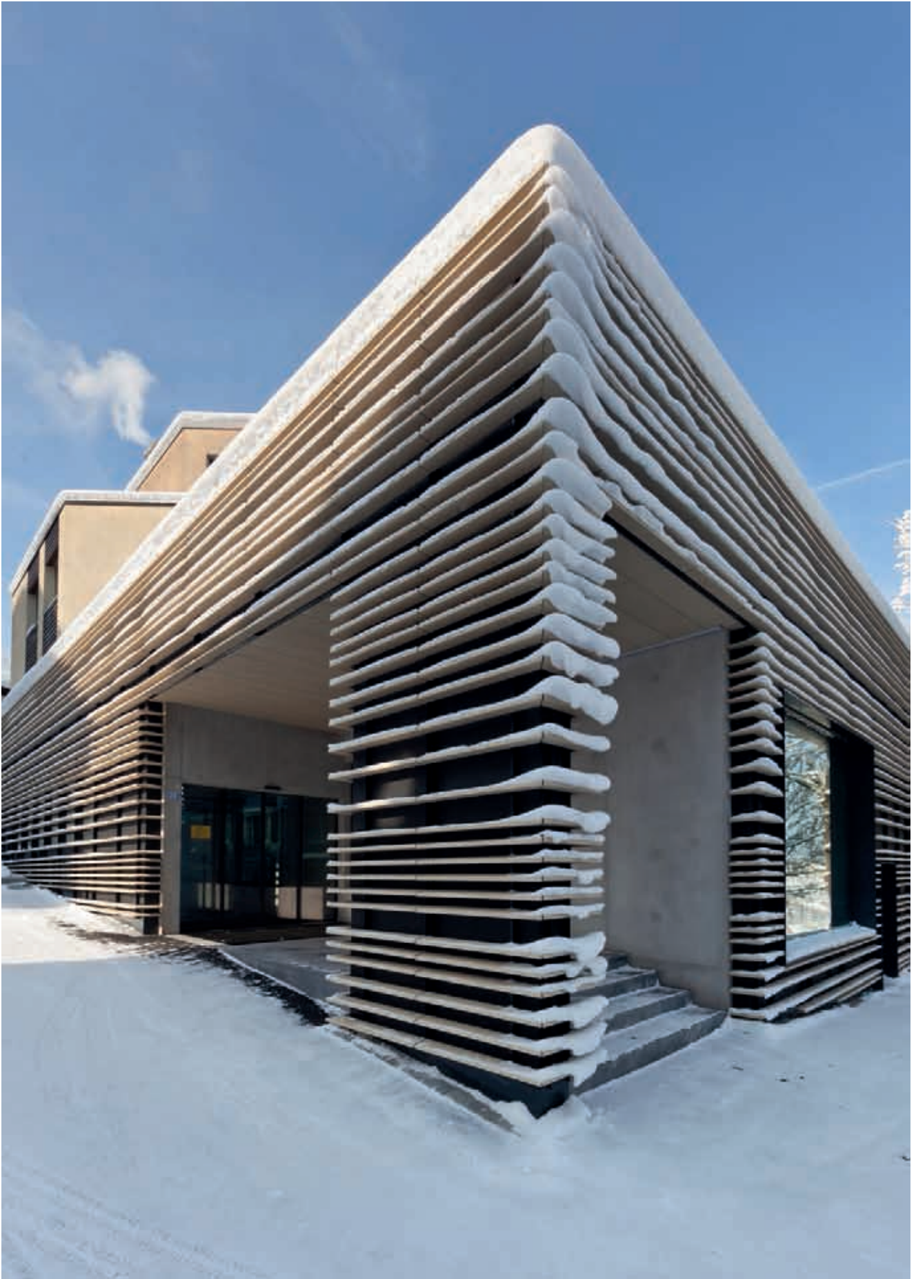
What may look like baguettes are actually NBK TERRART® Solid elements installed lying on their sides to create the visual impression of rods or tubes. Positioned at varying distances, when viewed from further away the light terracotta strips resemble a stack of logs or tree rings; however, on closer inspection they reveal themselves to be an open structure that allows the viewer to see the load supporting profiles and the dark skin of the facade. The three-dimensional design creates amazing impressions throughout the changing seasons, with nature fleshing out the creative design with additional meaning.
