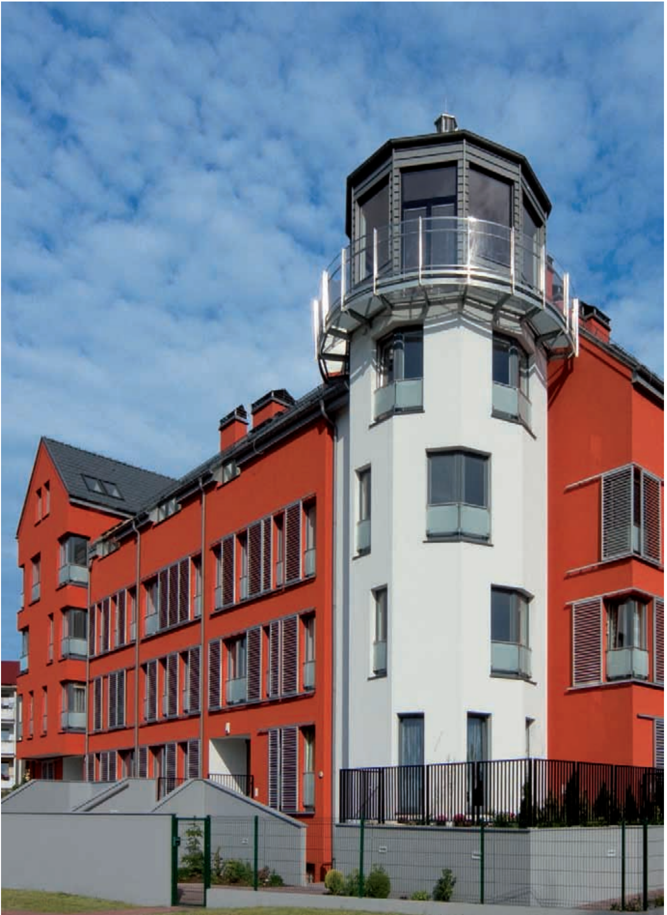
The Lighthouse Apartment is an attractive, 4 1/2 storey, multi-family residence building with an underground parking lot located in the town of Władysławowo. The building's tower was design in the style of a lighthouse, reflecting the Baltic sea traditions in the region. Project specific shutters provide striking façade details, ensuring light and heat regulation whilst providing privacy.
