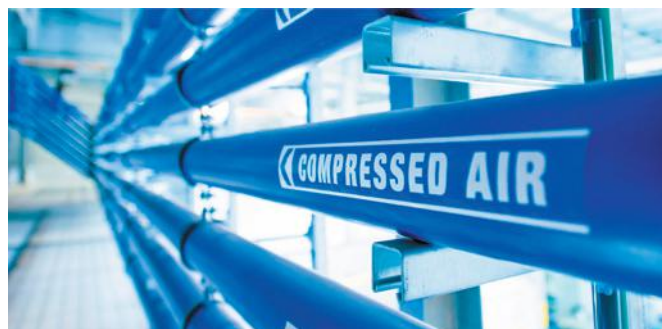
Image 3; The pipeline system should be laid in as many straight lines as possible to save energy.
