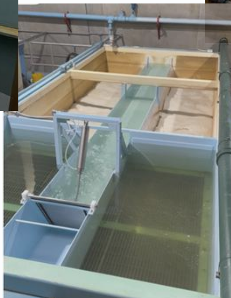
New filter trough gate
