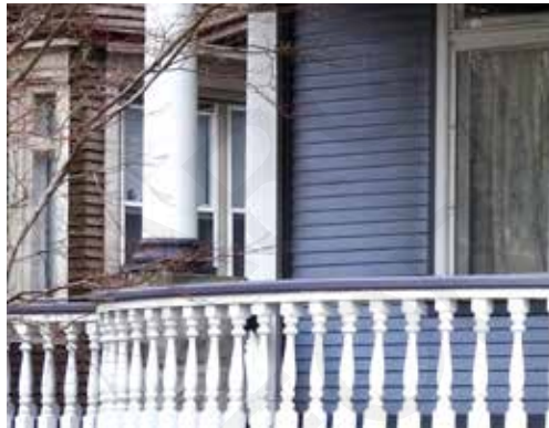
605 Richmond Avenue, detail
