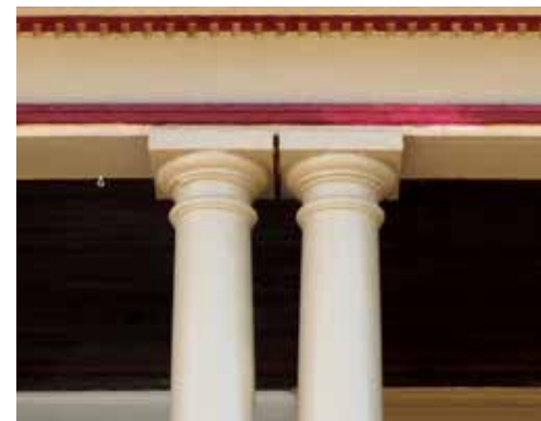
357 Ashland Avenue, detail
