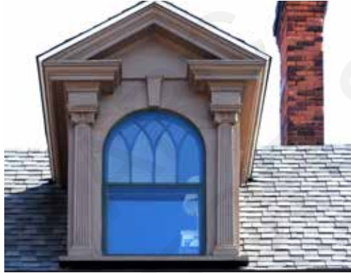
587 Ashland Avenue, detail
