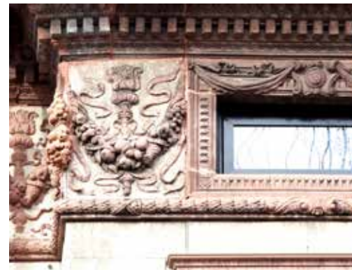
356 Richmond Avenue, detail
