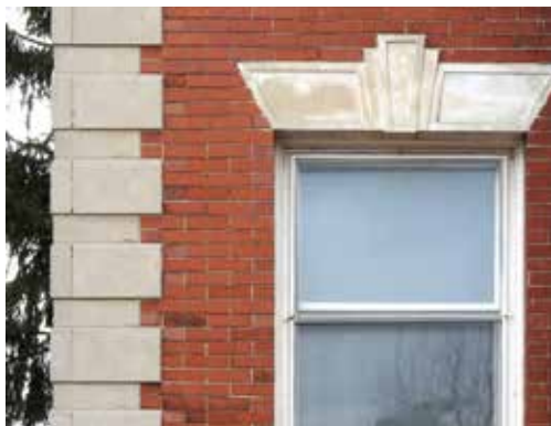
273 Richmond Avenue, detail
