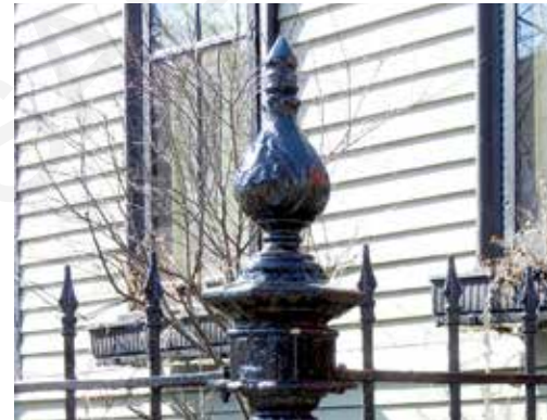
170 Ashland Avenue, detail
