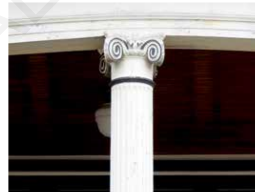
601 Richmond Avenue, detail
