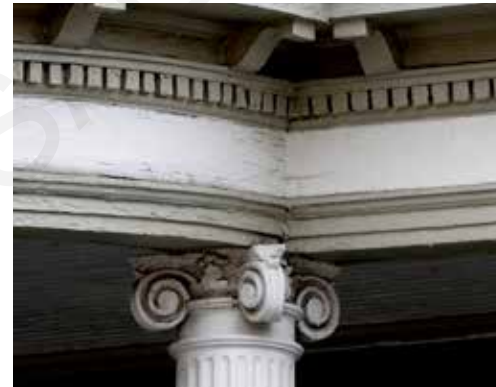
613 Richmond Avenue, detail
