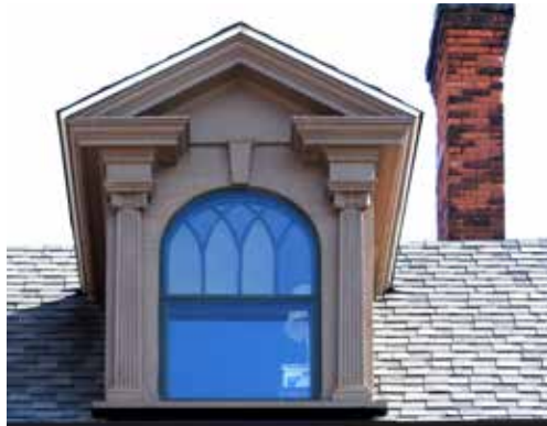
587 Ashland Avenue, detail
