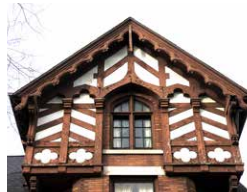
460 Richmond Avenue, detail
