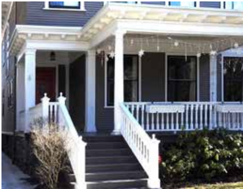
603 Richmond Avenue, detail
