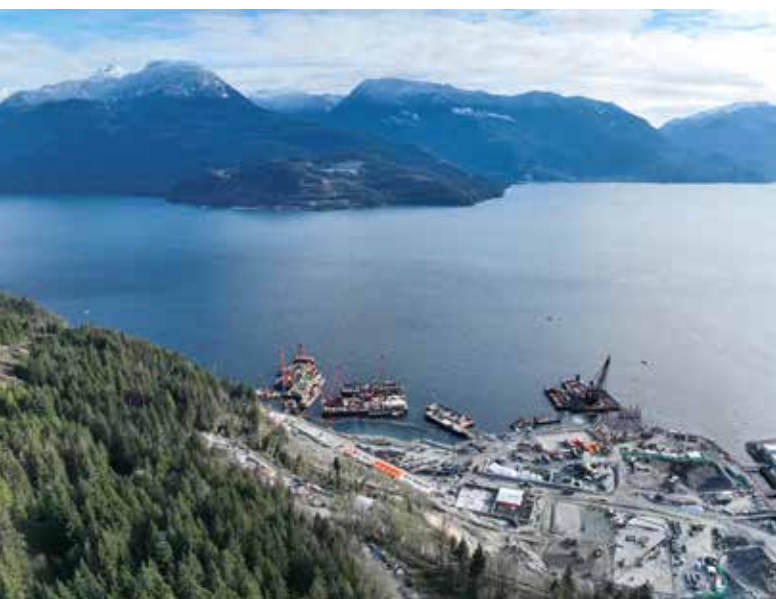
Construction in the Howe Sound, British Columbia.
