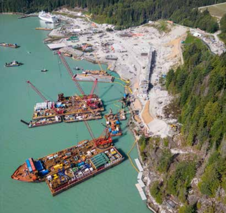
Construction work and access on the water.
