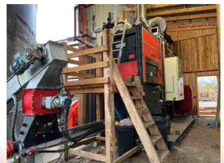
Biomass boiler system
