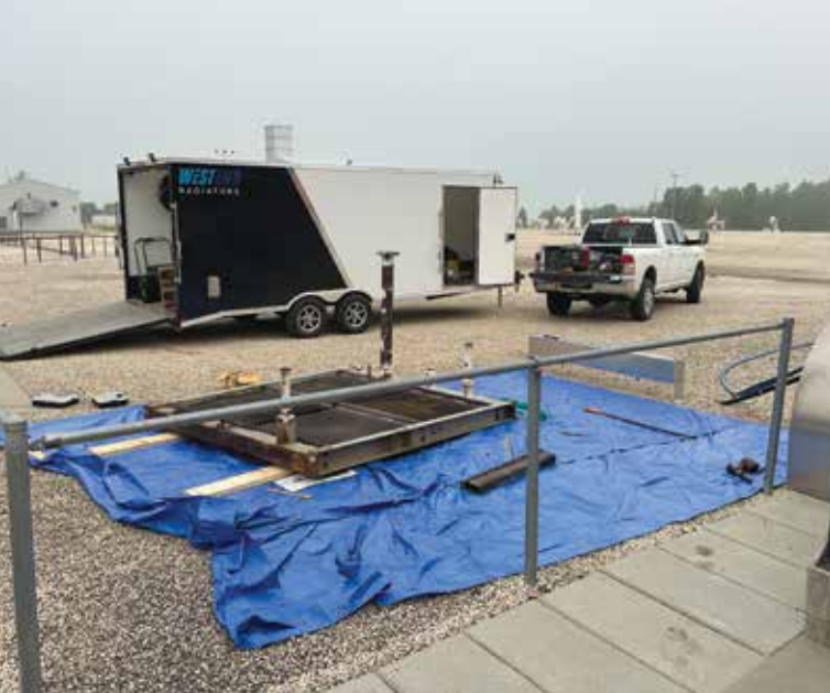
West End Radiators' mobile technicians repair a back-up generator heat exchanger on-site at a compressor station in Saskatchewan.
