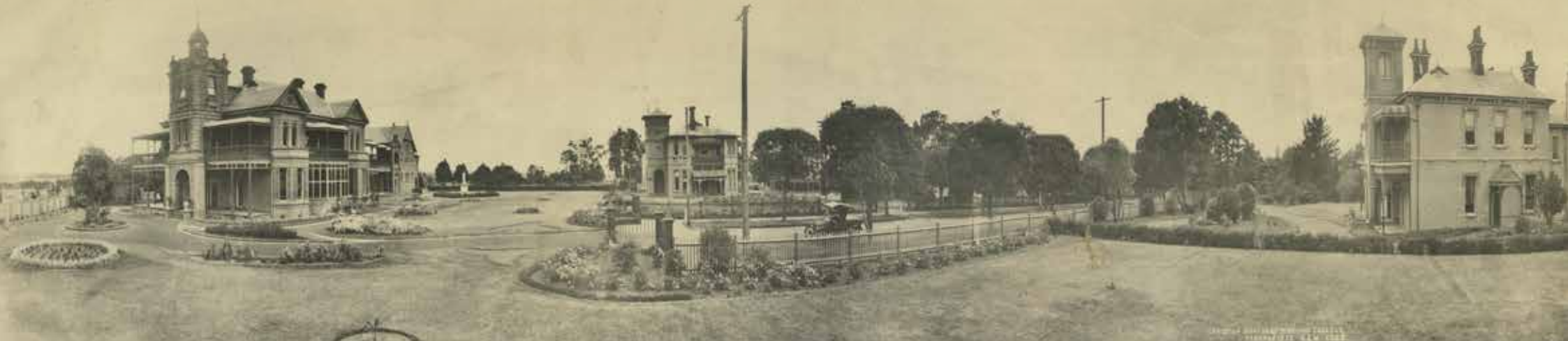
Albert Road, Strathfield, 1922 showing, from left: Mount Royal , Ovalau and Andross , Strathfield Local Studies
