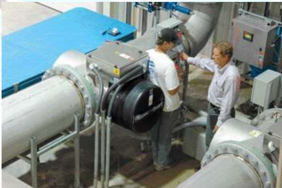
Arrow Creek Ultra Violet Disinfection Equipment
