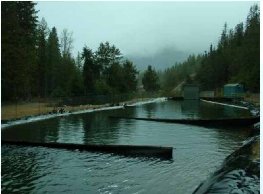
Arrow Creek Raw Water Supply
