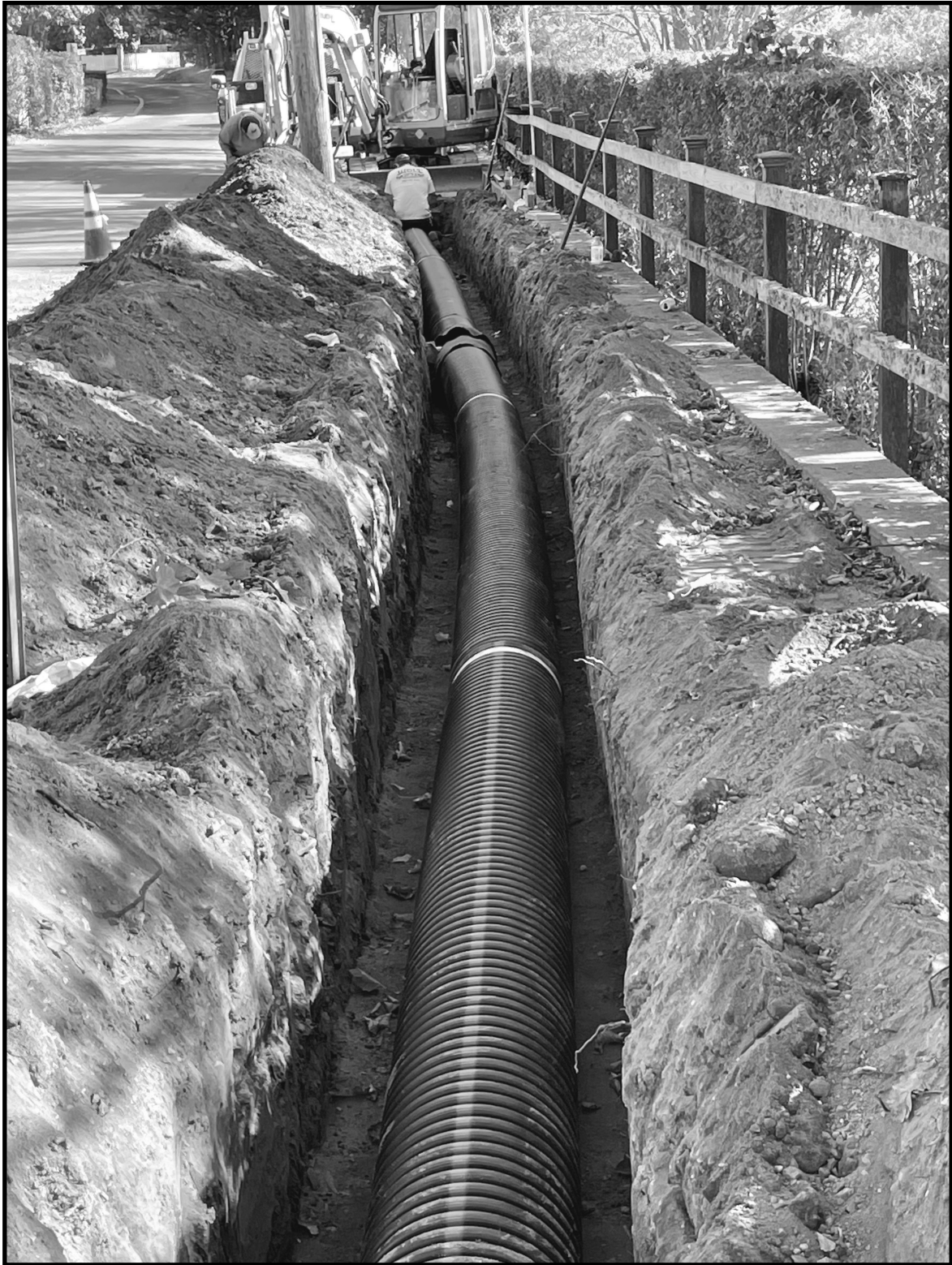
Installing new street drain pipe on Pease's Point Way North.
